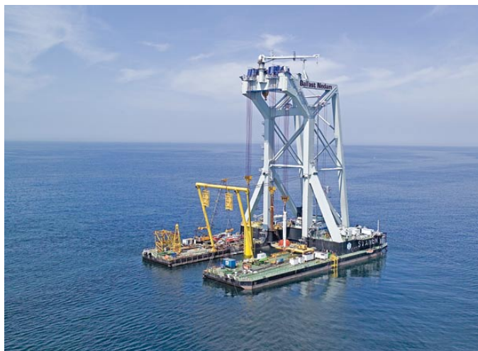
Crane barge "Svanen" - installation of transition piece.
