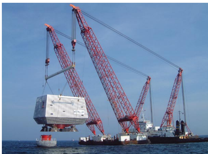
Crane barge "Rambiz" - installation of offshore sub-station.
