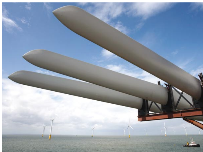
Three 52m long blades awaiting installation.
